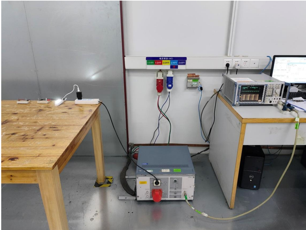
Conducted emissions from the AC mains power ports
